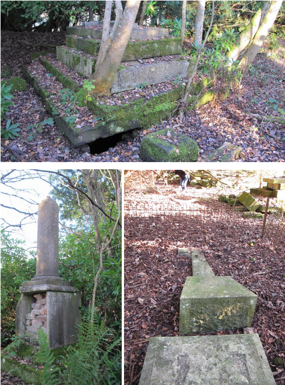
Fig 47. Clockwise from top - Examples of invasive tree growth, toppled gravestone, and vandalism to the 5 th Earls gravestone within St. Andrew's Chapel graveyard
