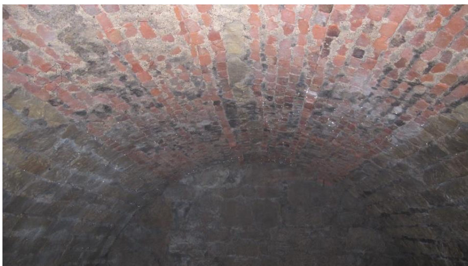
Fig 35. Barrel vaulted roof to icehouse
