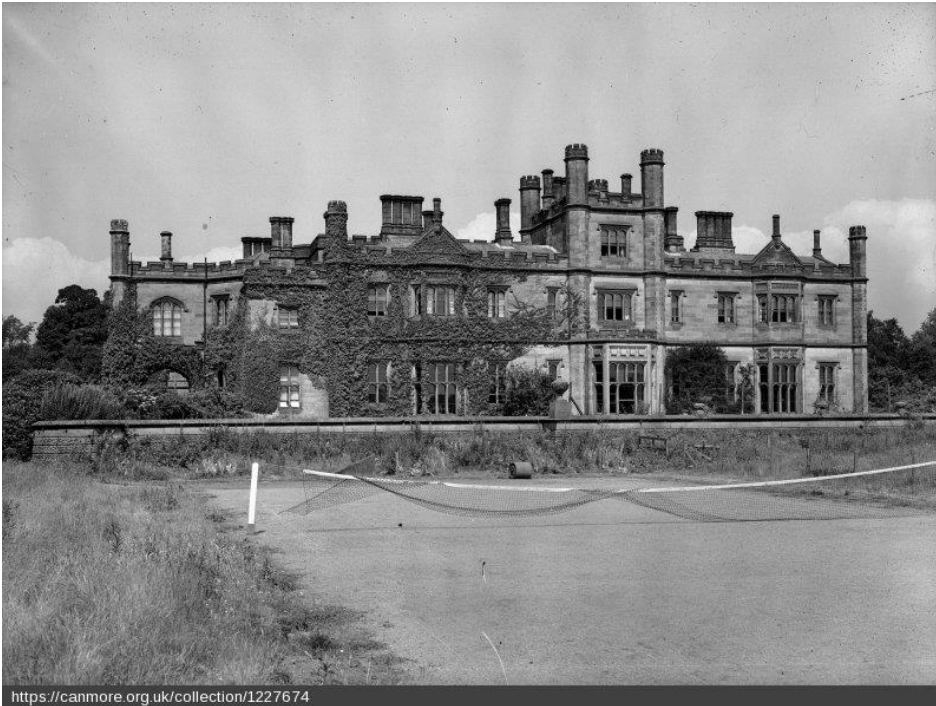
Fig 20. Principle south façade and terrace from oblique angle dated 1960. Copyright courtesy of HES (Scottish National Building Records)
