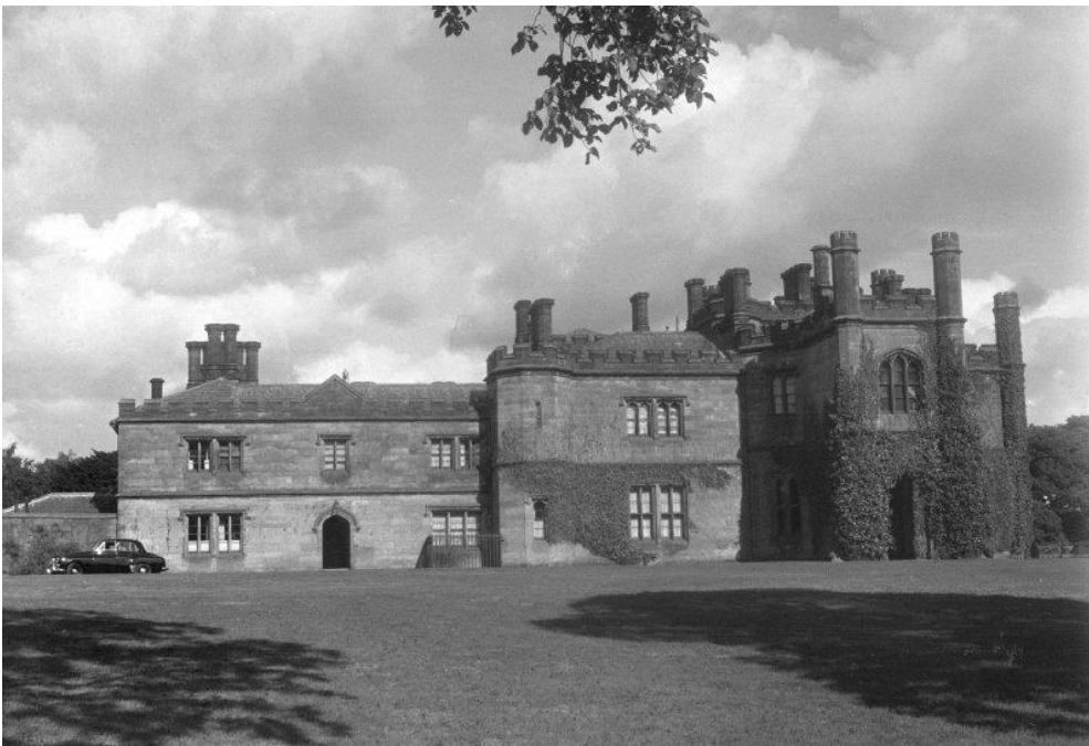
Fig 21. West façade including porte-cochere entrance dated 1955. Copyright courtesy of HES (Scottish National Building Records)
